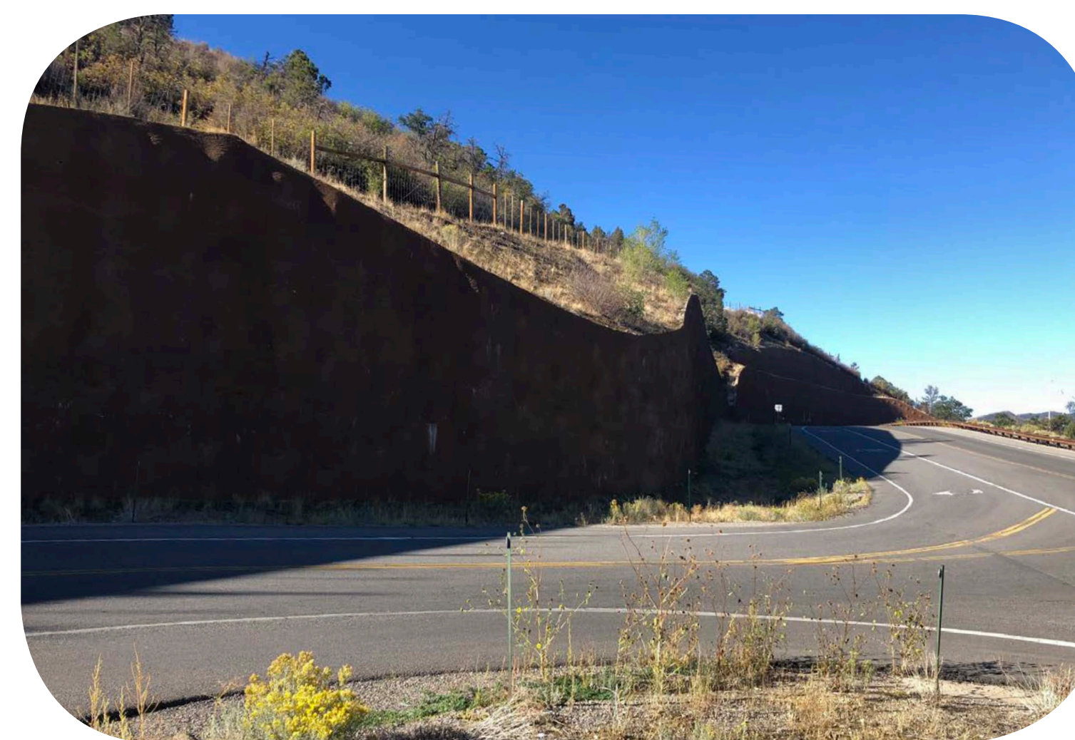
Wall to be removed at US 550 and US 160
